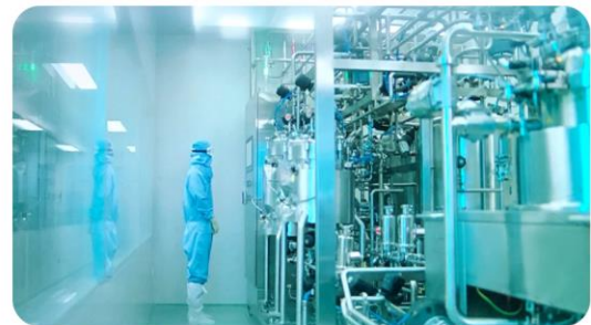
Dedicated production equipment installed in our factory
